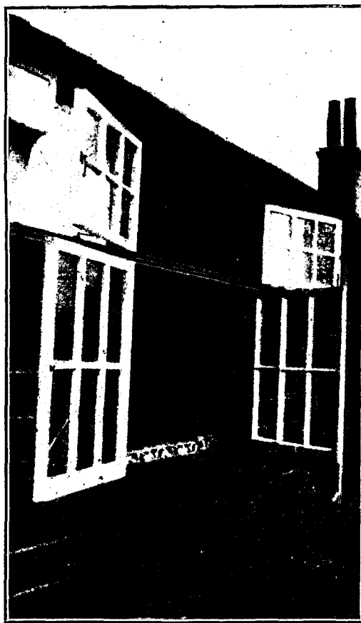
Windows Opening Outwards, Sanatorium Pattern.
